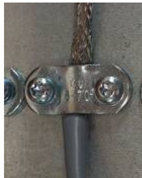
PE clamp connection for cable shield (max 2.5 Nm)
