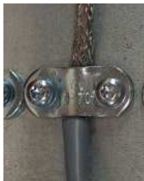
PE clamp connection for cable shield (max 2.5 Nm)
